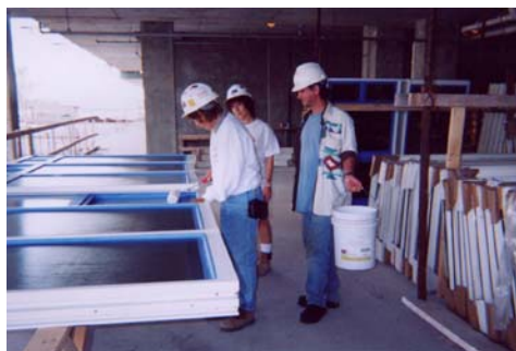
Cortec® MCI® Peel Off Coating protects glass windows from construction debris while significantly reducing time and labor costs.
